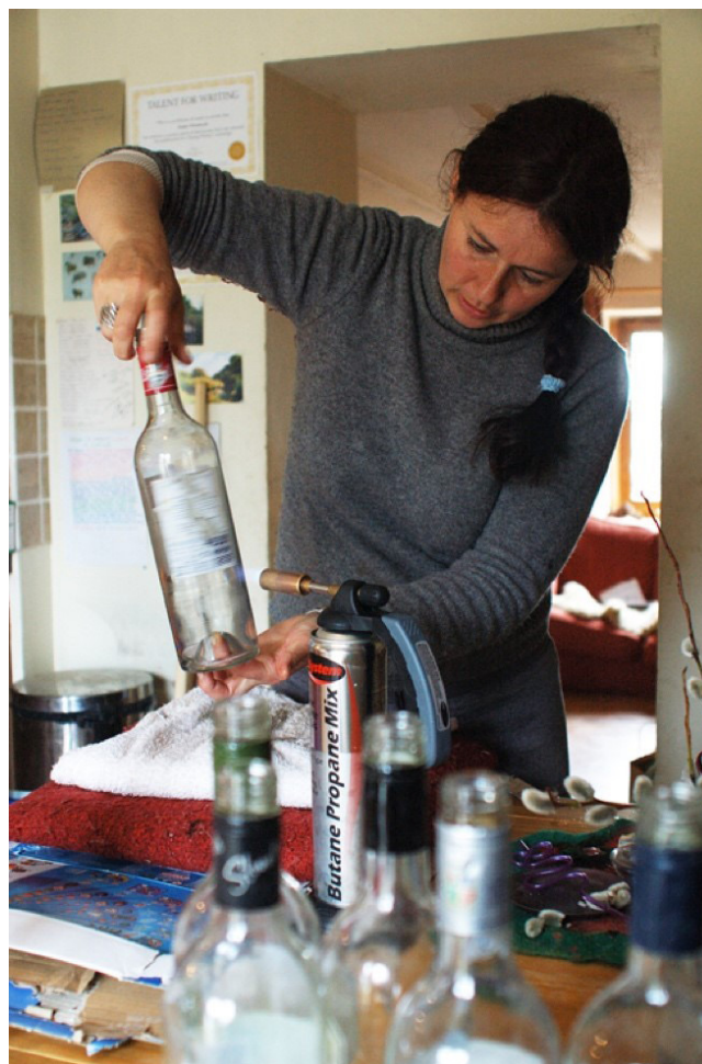
Hoppie cutting old wine bottles into glass bricks for use in the construction of a wall in her eco-house
